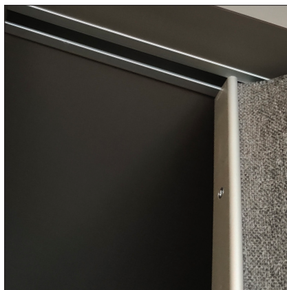
Ceiling profile embedded in ceiling.
